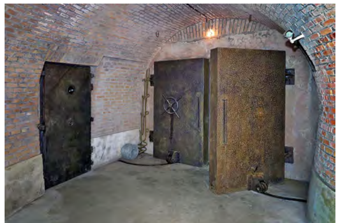
Villa Ada main entrance blast doors. The small door to the left leads to a guard room
